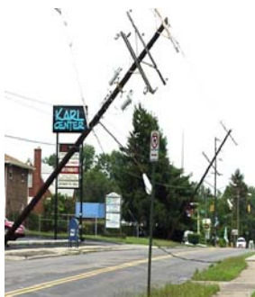
Northridge Rd. and Karl Rd. on 8/9/2000
